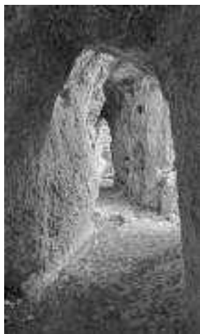
38. Tunnel of a 25 km Roman aqueduct built in the 1st century near Albarracín ©Diego Delso
