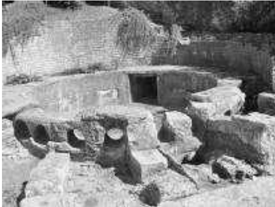
39. Urban distribution depot in Nîmes, France. The circular section pipes leave from a central reservoir, fed by a square section aqueduct. ©Przemysław Sakrajda
